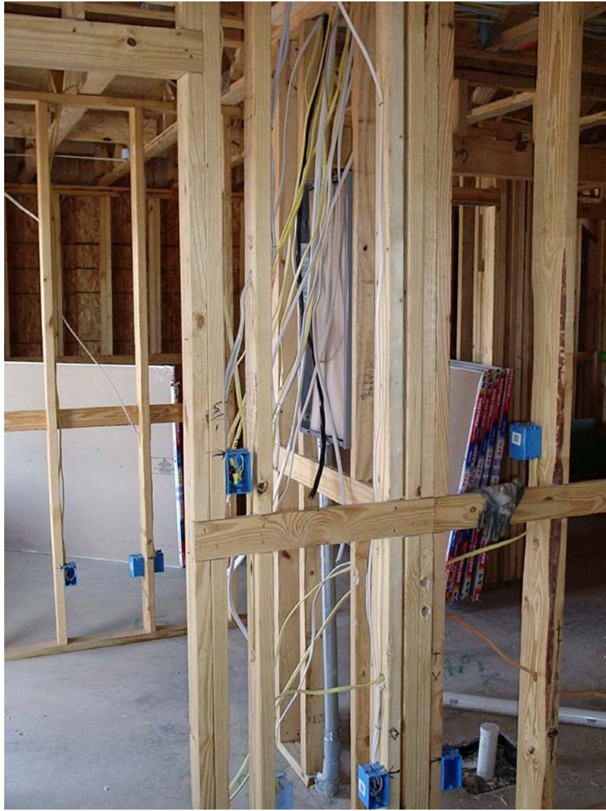
BLOCK 'B' - BUILDING 14 Wiring To Electrical Panel W/ Sheetrock in Background
