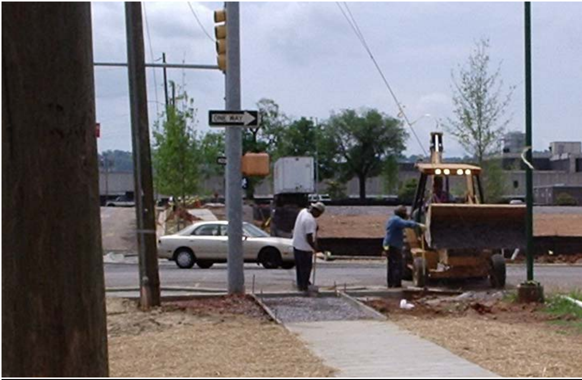
SIDEWALK CORNER WORK Intersection of 6 th Avenue & 25 th Street
