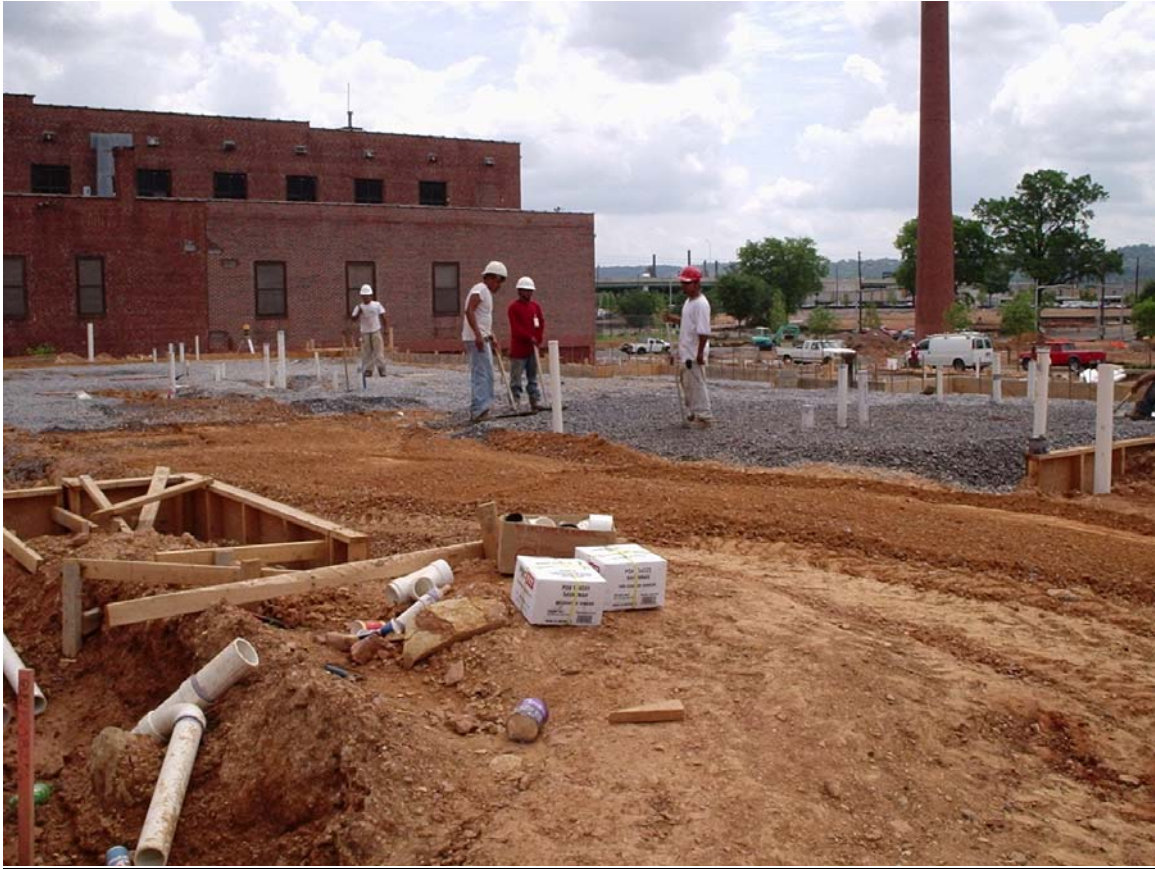
BLOCK 'C' NORTH - BUILDING 9 Underslab Work: Gravel, Plumbing Stubups
