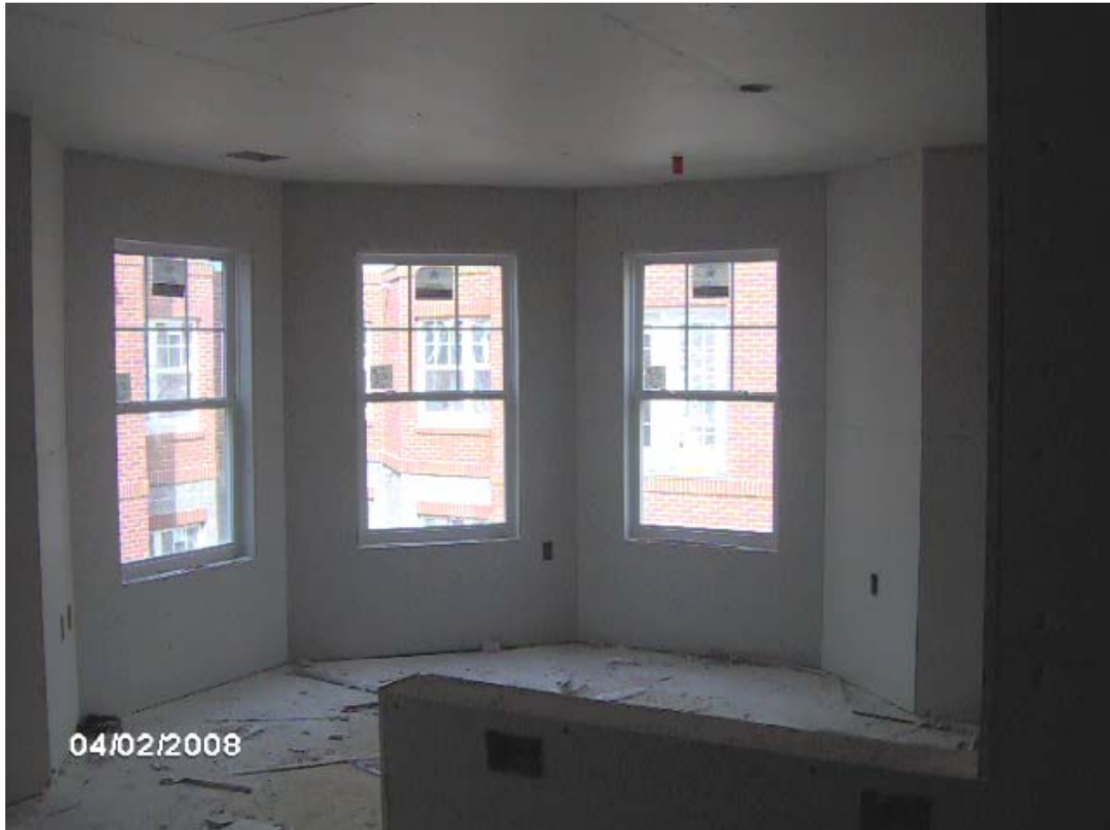
PARK PLACE - PHASE III Living Area of Interior Unit w/ Courtyard Beyond
