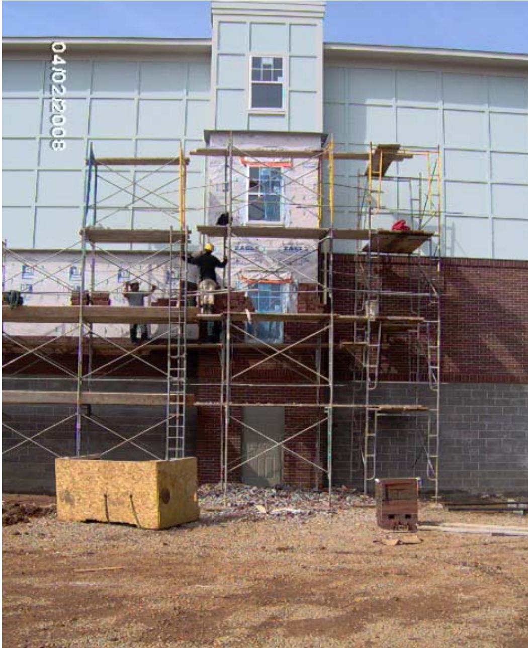
PARK PLACE - PHASE III Masonry Installations
