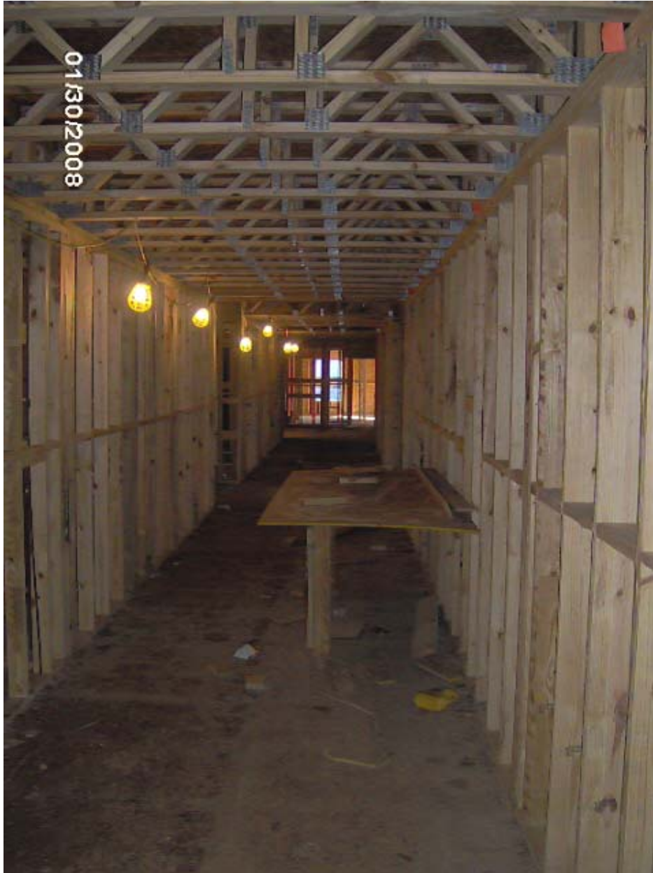
PARK PLACE - PHASE III Framed Interior Corridor
