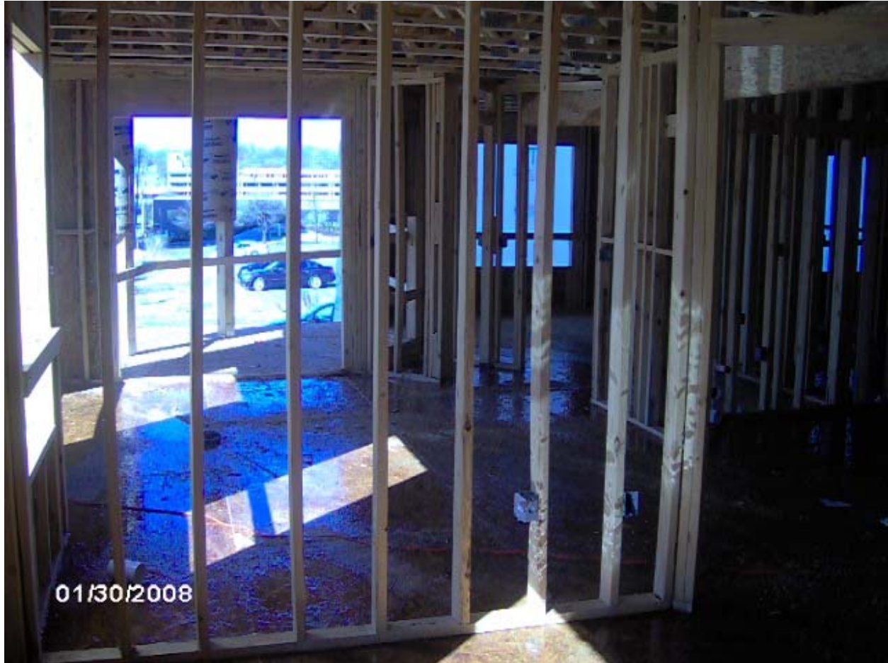
PARK PLACE - PHASE III Interior Partition Framing with Corner Balcony Beyond
