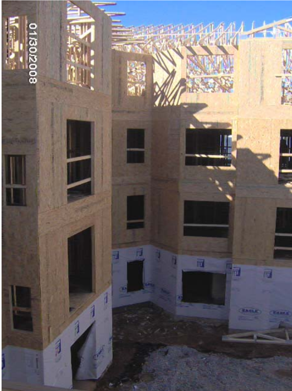
PARK PLACE - PHASE III Framing @ Interior Courtyard Area
