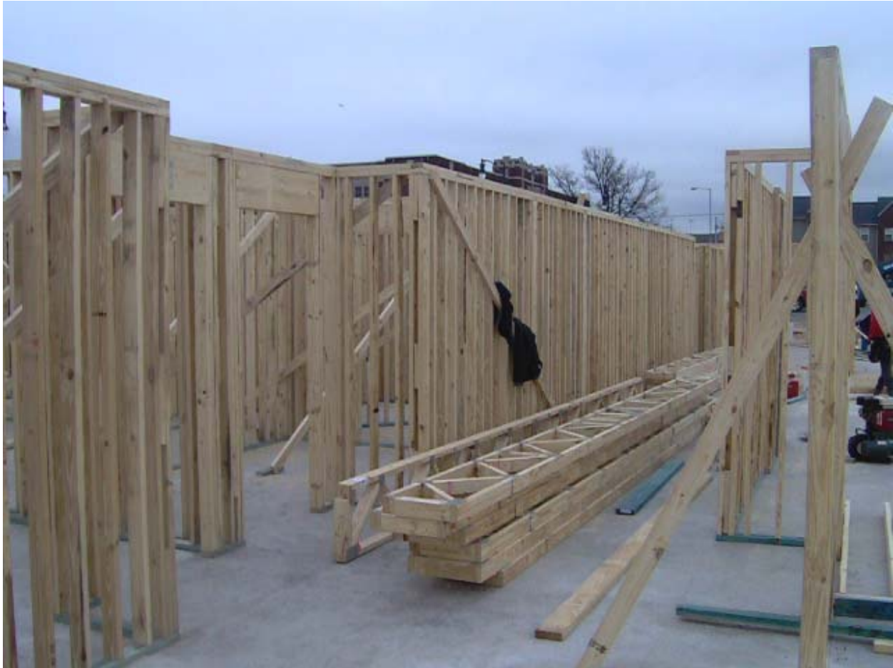
PARK PLACE - PHASE III First Floor Wall Framing
