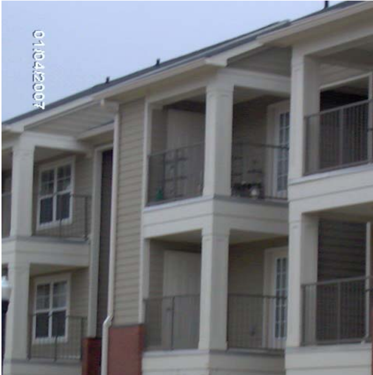
BLOCK 'F' – BUILDING 3 Tenant Items on Balcony
