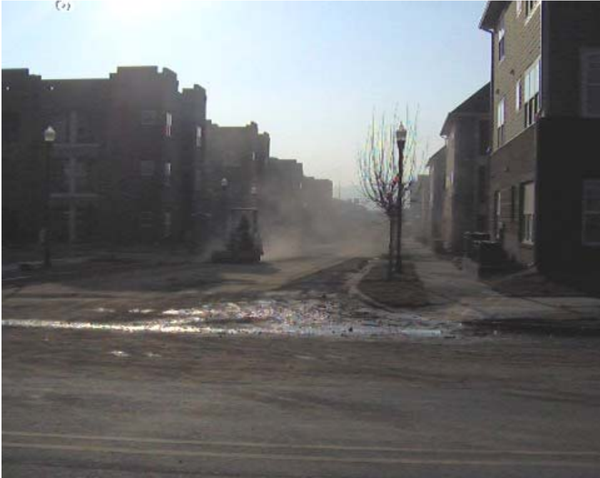
BLOCK 'D' – GREEN STREET Street Cleaning
