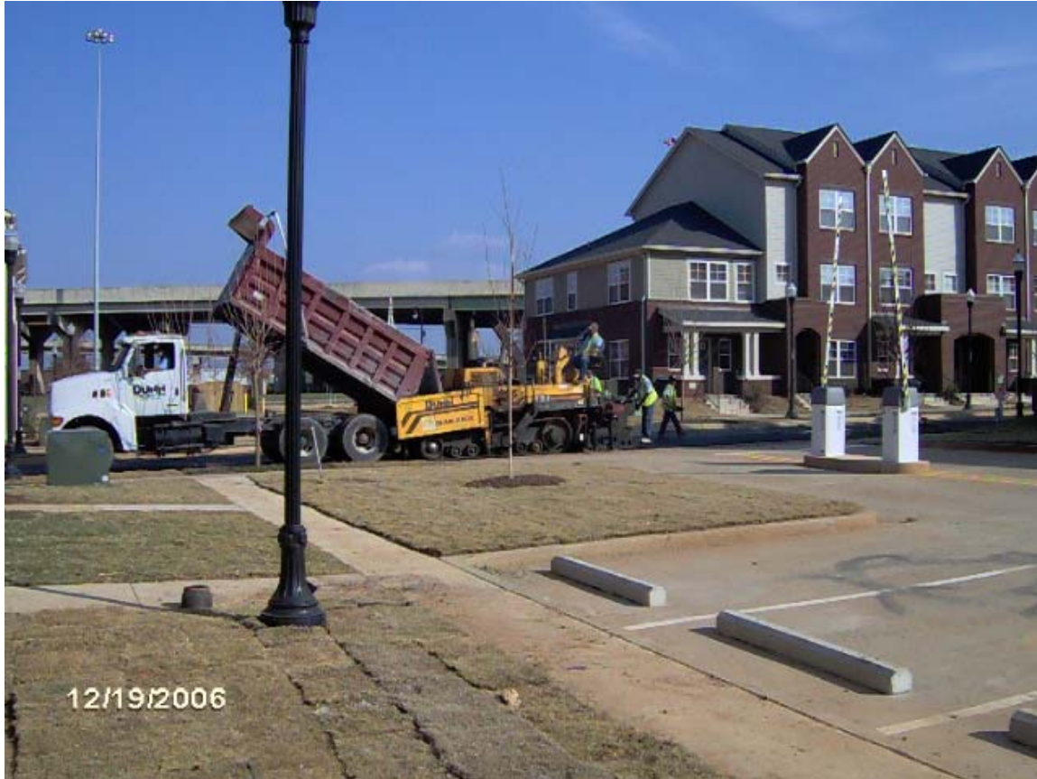
BLOCK 'E' – GREEN STREET Asphalting Of Street
