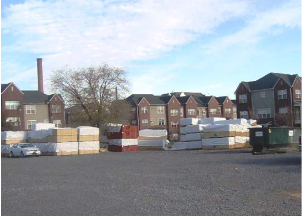
PARK PLACE - PHASE III On-Site Stored Materials
