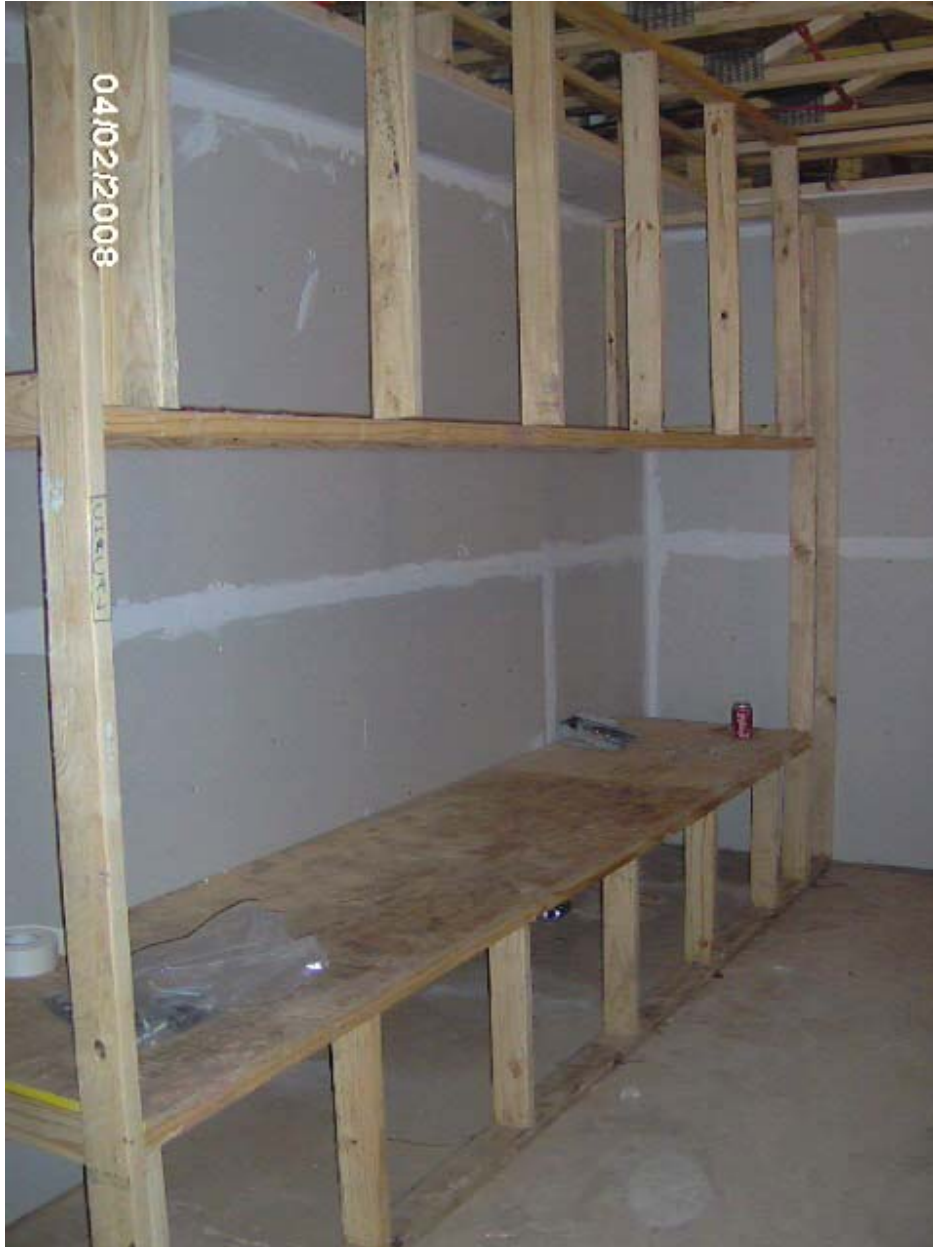
PARK PLACE - PHASE III Framing at Lower Level for Mailboxes
